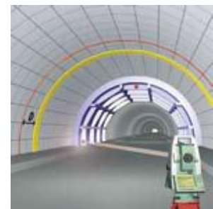
Spot-on positioning of the arch formwork and setting out joint strips
